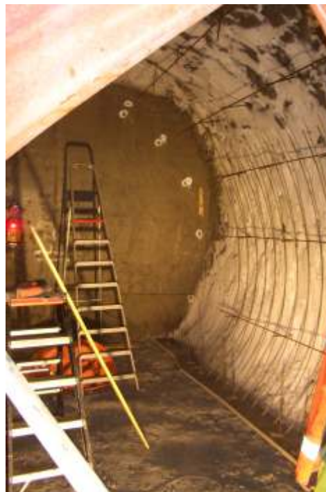
Excavated Cross Passage with exposed frozen walls
