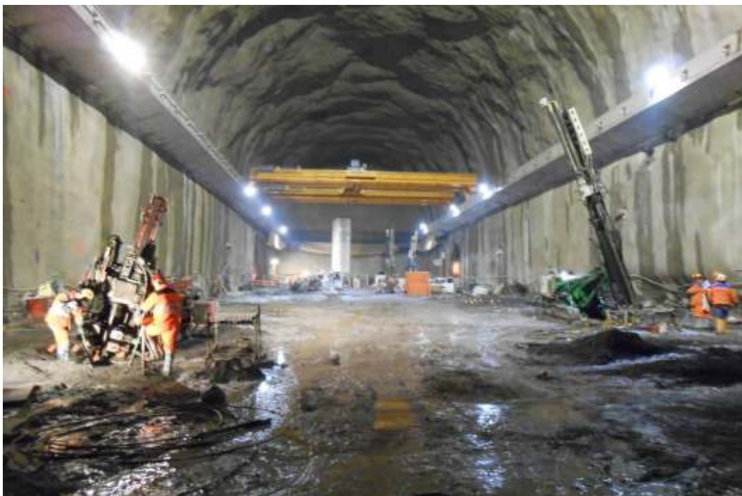
Drill rigs in work in the main cavern
