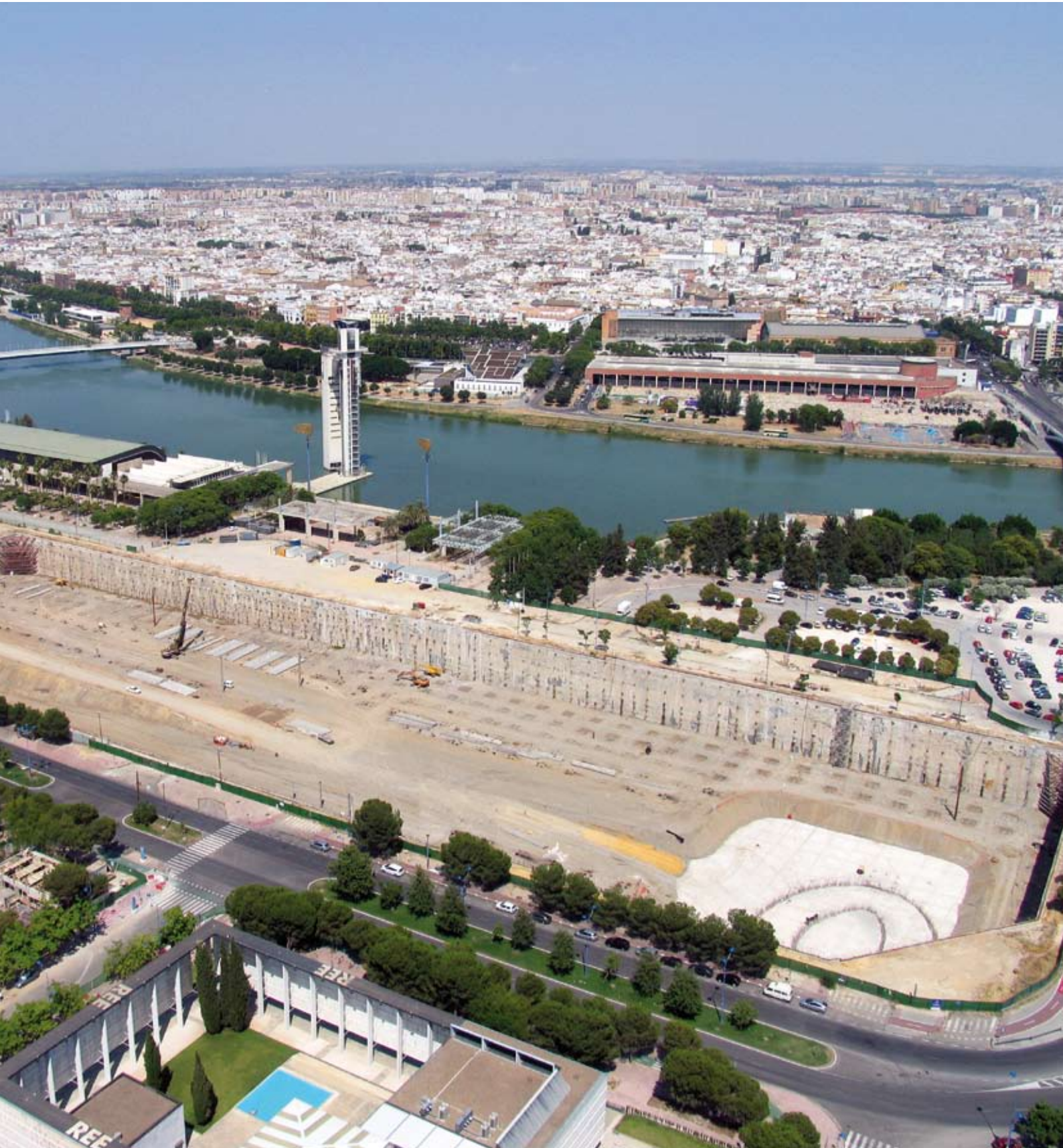
Foundation and Diaphragm walls in Torre Cajasol Project. Sevilla Diaphragm walls
