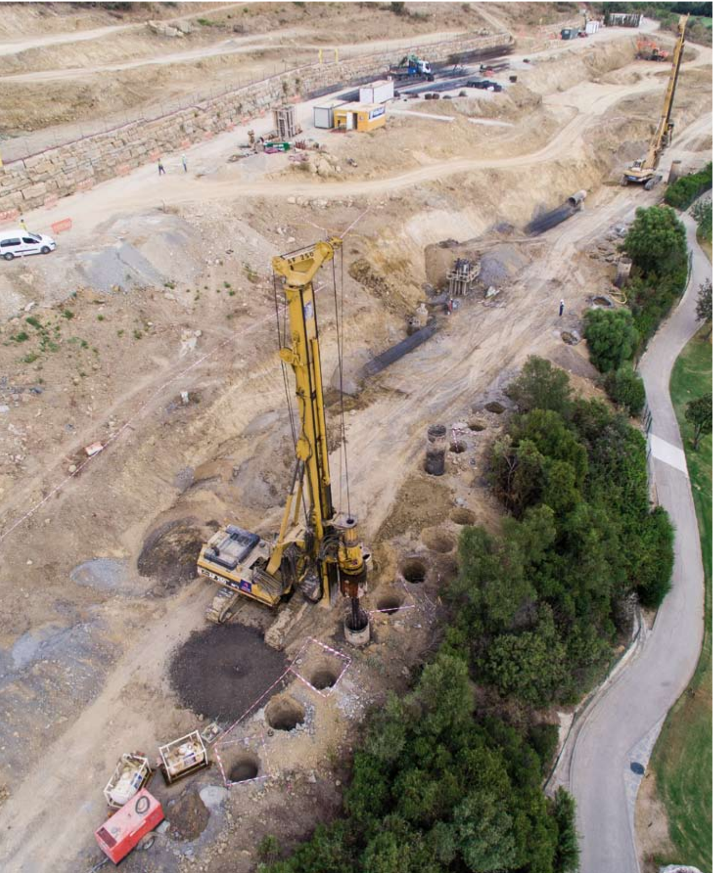
Slope stabilization for construction of 15 Villas in Finca Cortesín. Casares. Malaga, Spain Bored Piles
