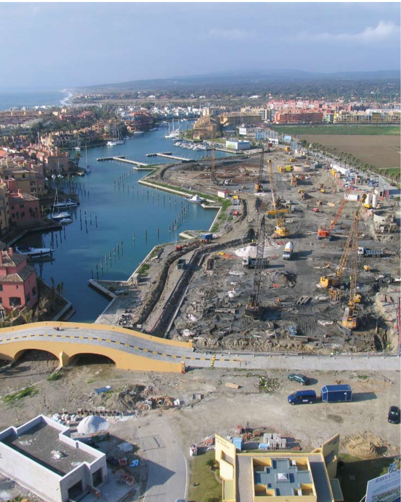
Residential Building Sotogrande, Cádiz, Spain Diaphragm walls
