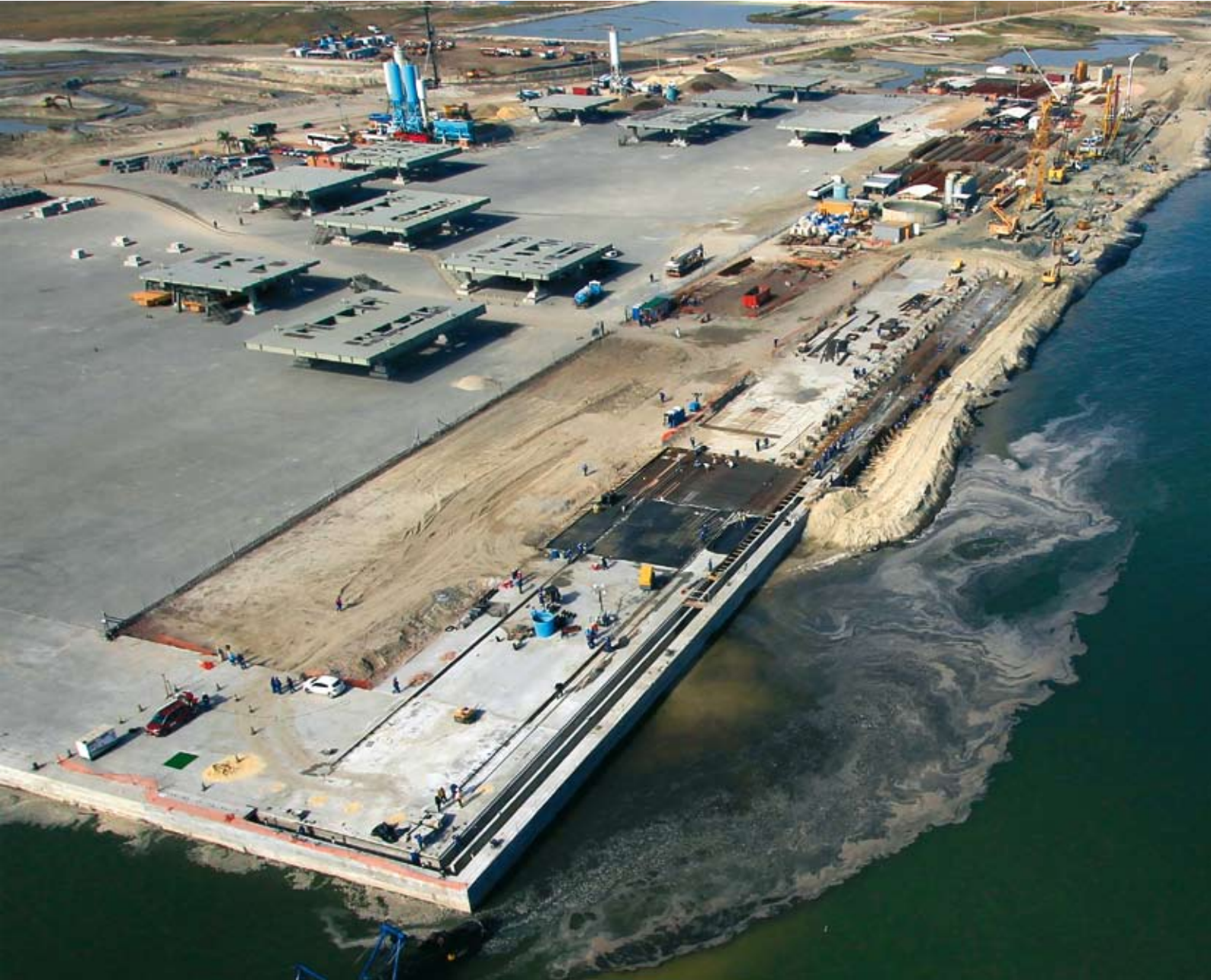
Açu Port, Brazil Diaphragm walls
