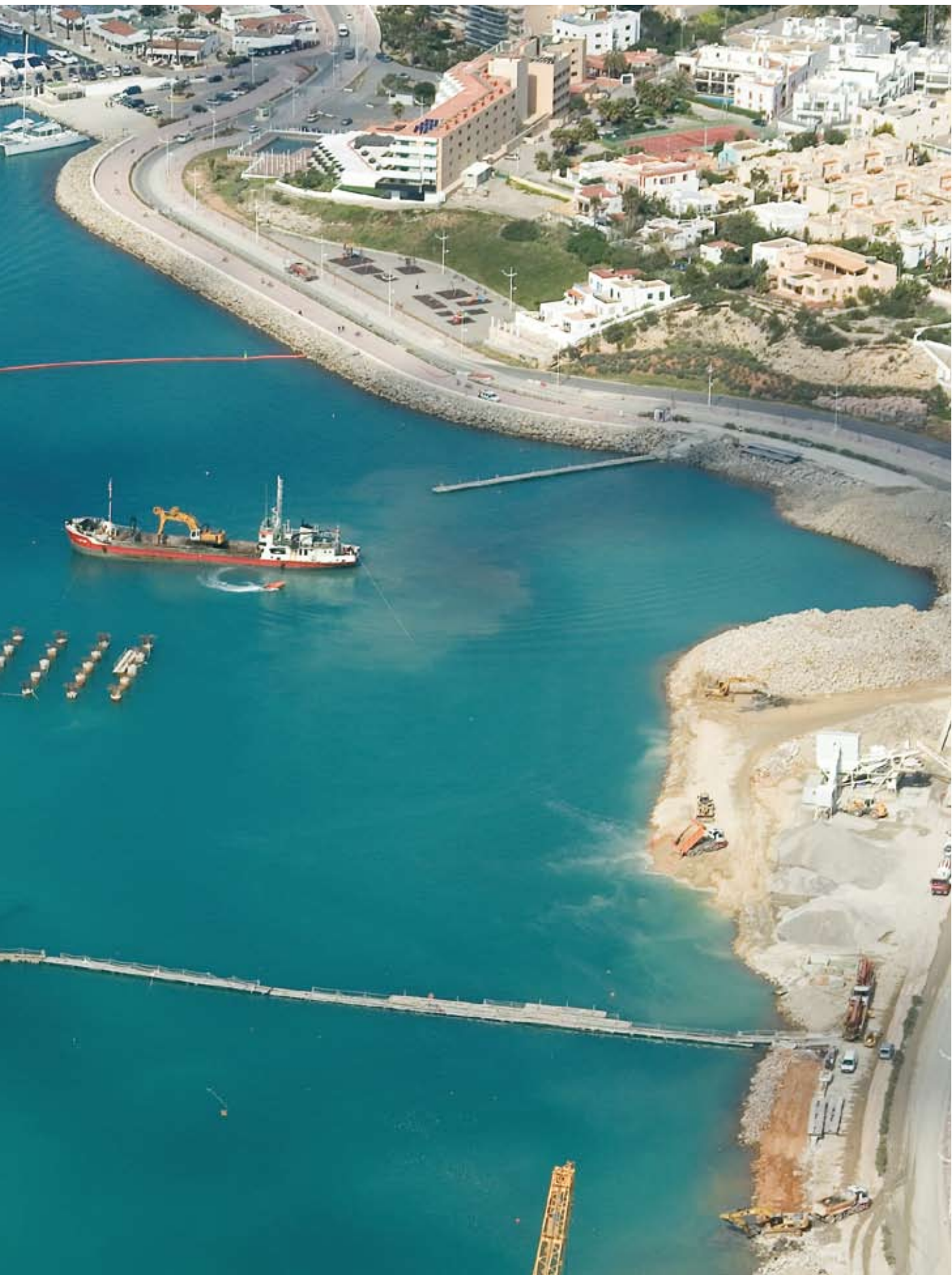
Botafoc Pier. Ibiza Port, Spain Bored Piles
