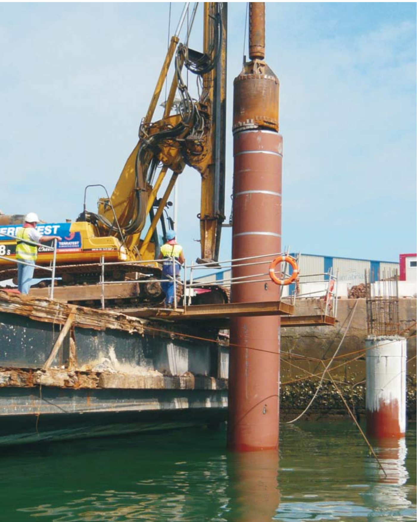
Bridge Foundation in Maliaño Pier, Santander Port, Spain Bored Piles
