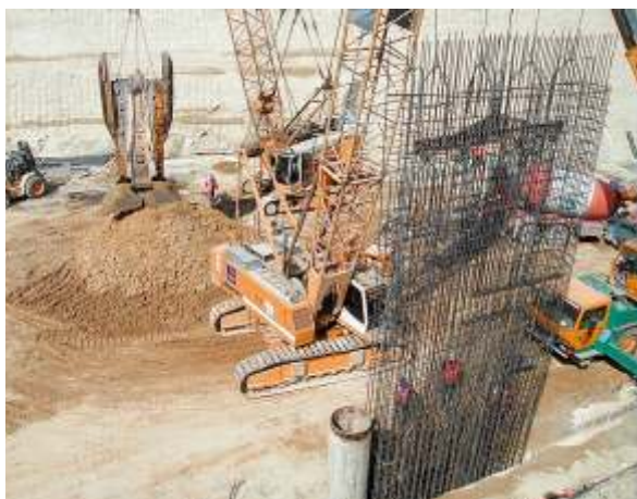
Armed and concrete placement through tremie pipe
