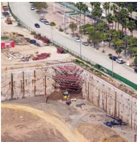
Strut diaphragm walls using metal structures and anchors
