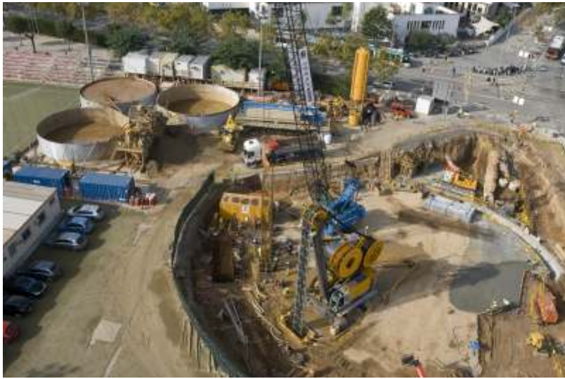
Diaphragm Walls with Trench-Cutter for Barcelona Metro Line 9 Pozos Station
