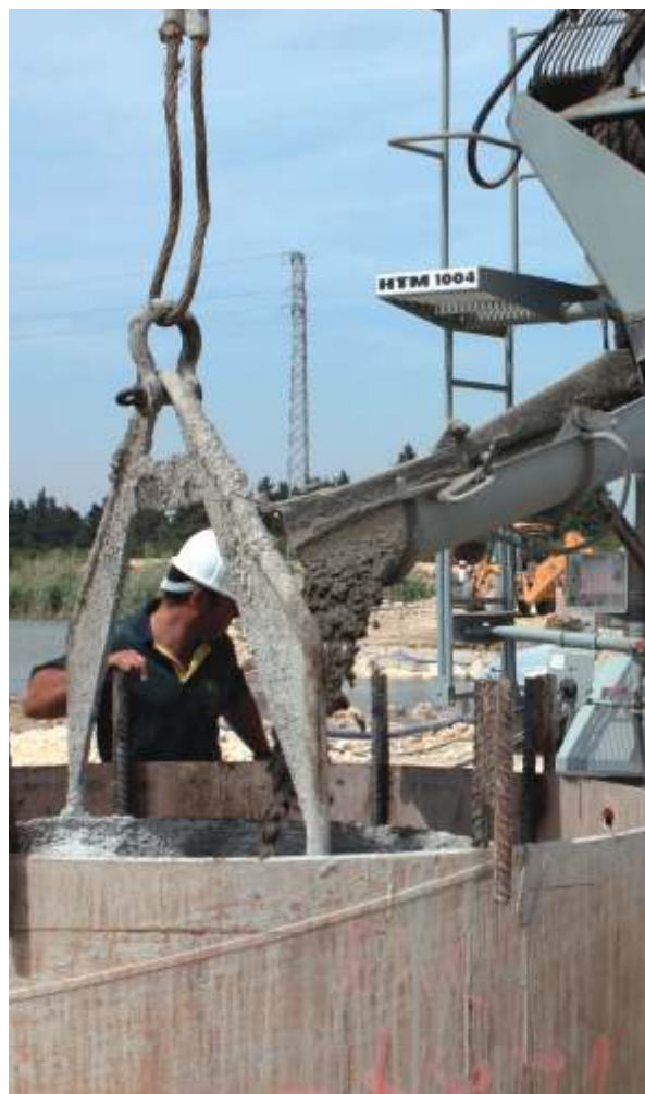
Concreting piles using tremie tube
