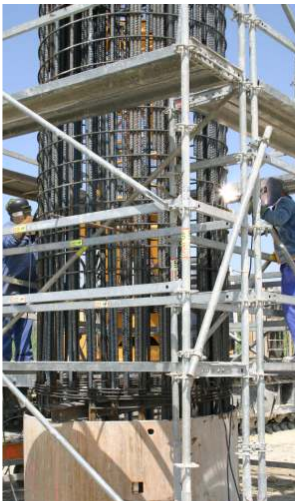
Overlapping and fitting of pile reinforcement
