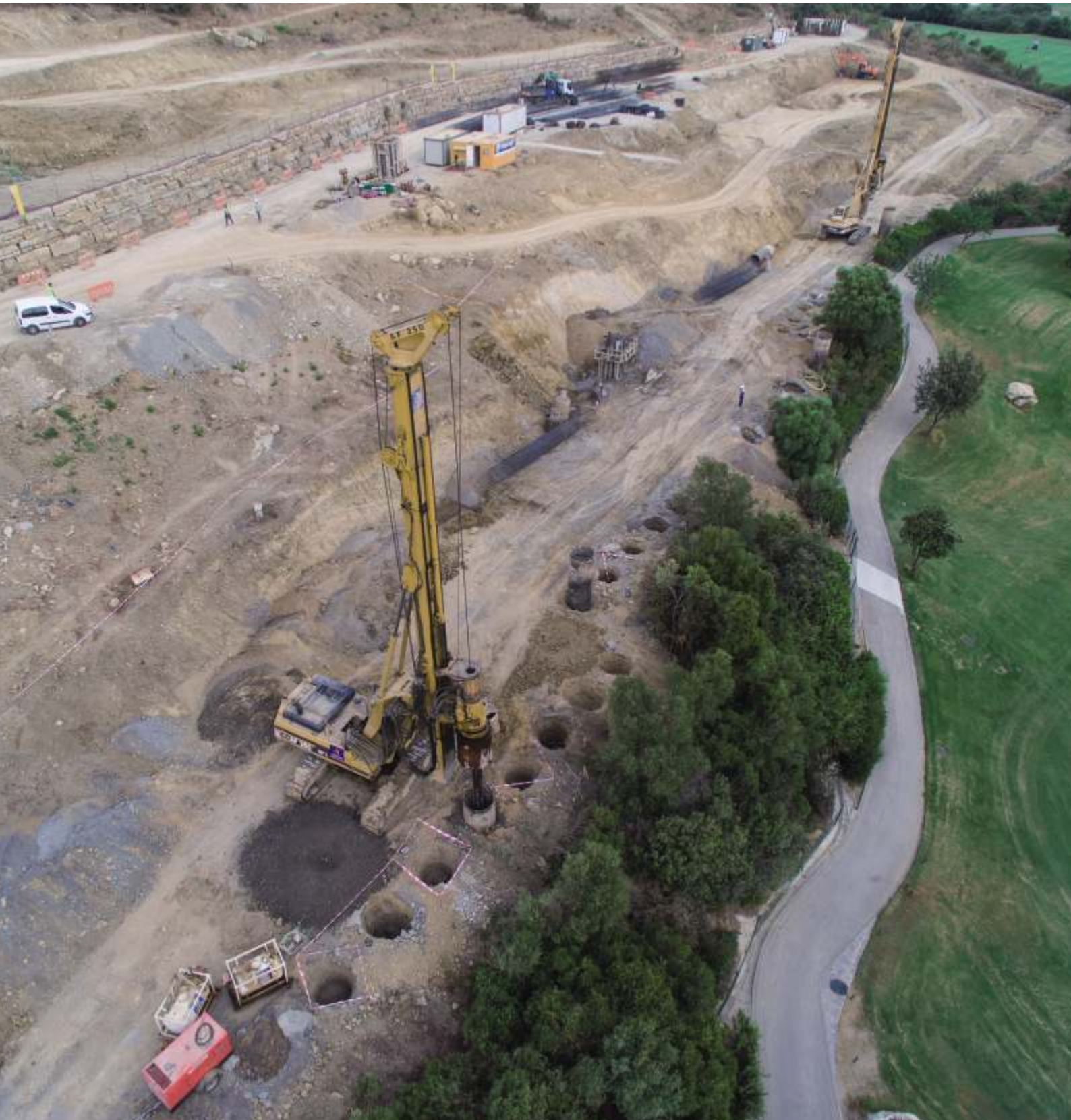
Slope stabilization for construction of 15 Villas in Finca Cortesín. Casares, Malaga, Spain
