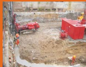
Jet Grouting. Victoria Center- București
