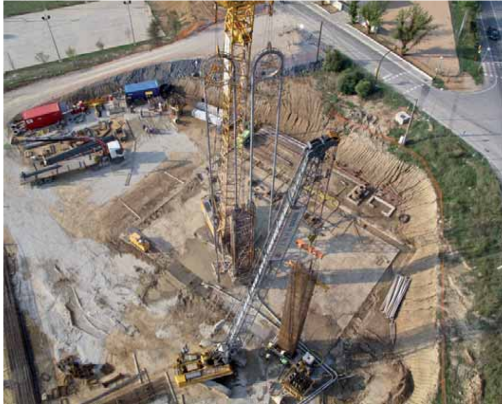
Santierul Sant Ponz, Gerona, Spania Trench cutter
