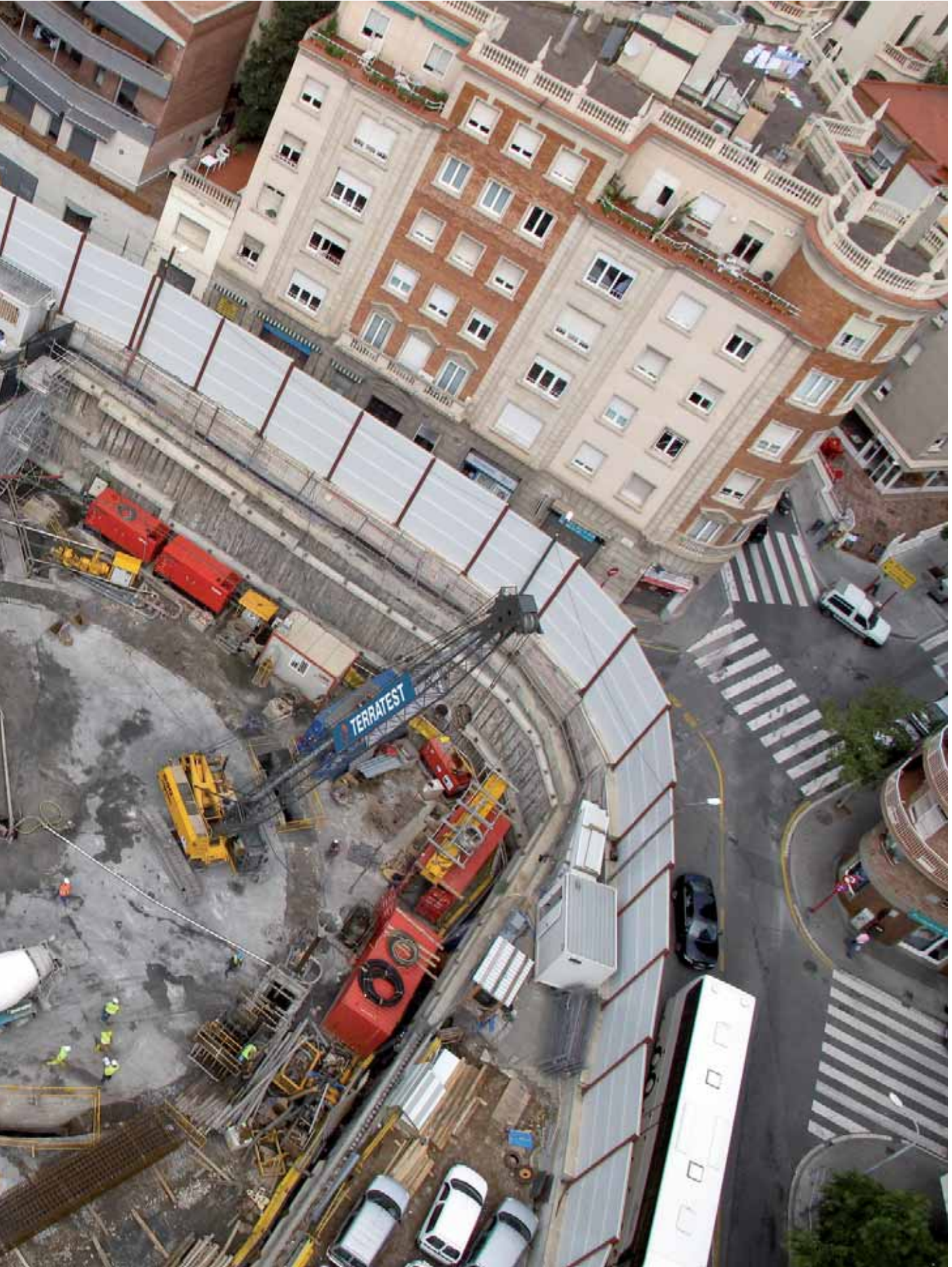
Metrou Barcelona, Linia 9. Plaza Sanllehy, Barcelona, Spania Trench Cutter
